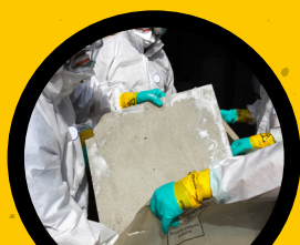
ASBESTOS MILLBOARD AND PAPERS
